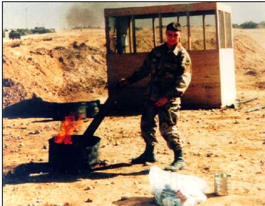
Figure B-7. Waste Burn-Out Activity with Latrine in Background Improvements to Burn-Out Latrine Technology are Shown in Figure B-8 Source: USACE, 2008
